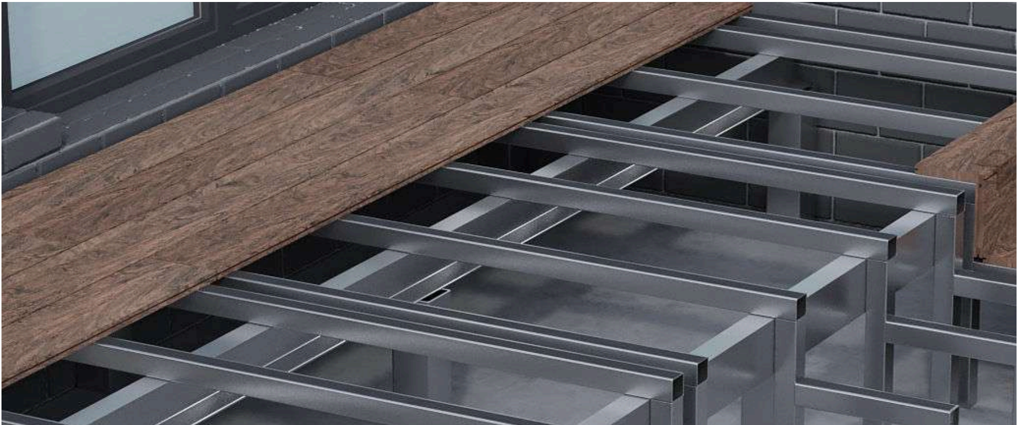
Metal frame installation.
